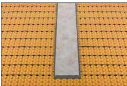
Joint sealing with Schlüter®-KERDI-KEBA
