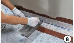
9. Apply a C2 adhesive on the membrane using the flat side of the notched trowel taking care to fill the circular cavities.10. Apply a C2 adhesive on the membrane with a notched trowel suitable with the size of the tiles and tiling.
