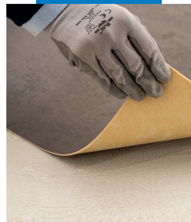
Installation of polyurethane-based flooring with Ultrabond Eco V4 Evolution
