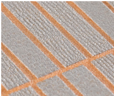
Finished Kerapoxy Easy Design 700 + Mapecolor Metallic Red Clay
