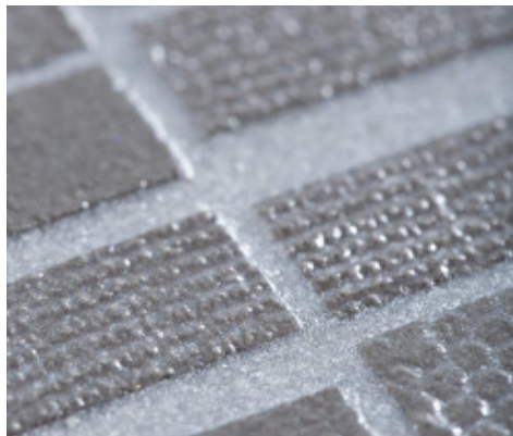
Finished Kerapoxy Easy Design 700 + Mapecolor Metallic Shining
