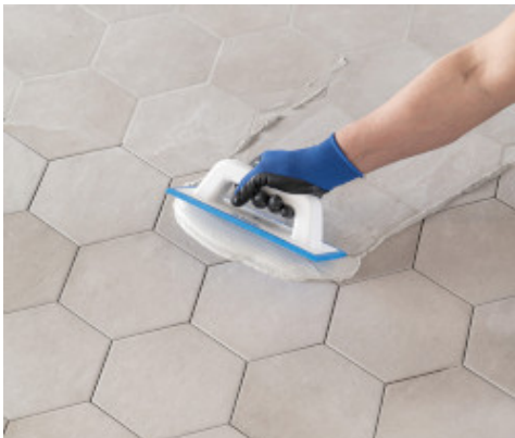
Application of Keracolor FF with MAPEI float
