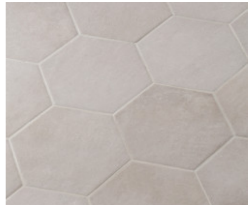
Floor grouted with Keracolor FF
